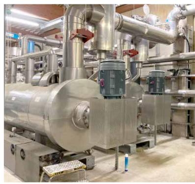
The thin-film dryers, above the droplet separator and to the right the insulated condensers. GIG Karasek
