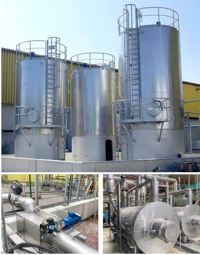
Pictured above: The foundation and masonry of the tank farm were constructed by Power Oil, while the tanks, supports, and piping were built by GIG Karasek. Picture at left: Sampling point. Picture at right: The blue lubricant cartridge for lubricating the bearings is easy to replace and only needs to be changed twice a year. © GIG Karasek
