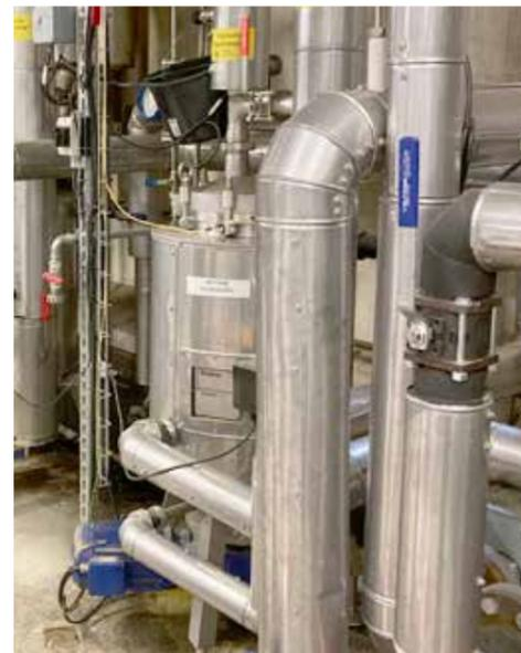
Pictured above: Pipe with sight glass to check the lecithin, and underneath, the pump to convey it to the rear to the coolers.
