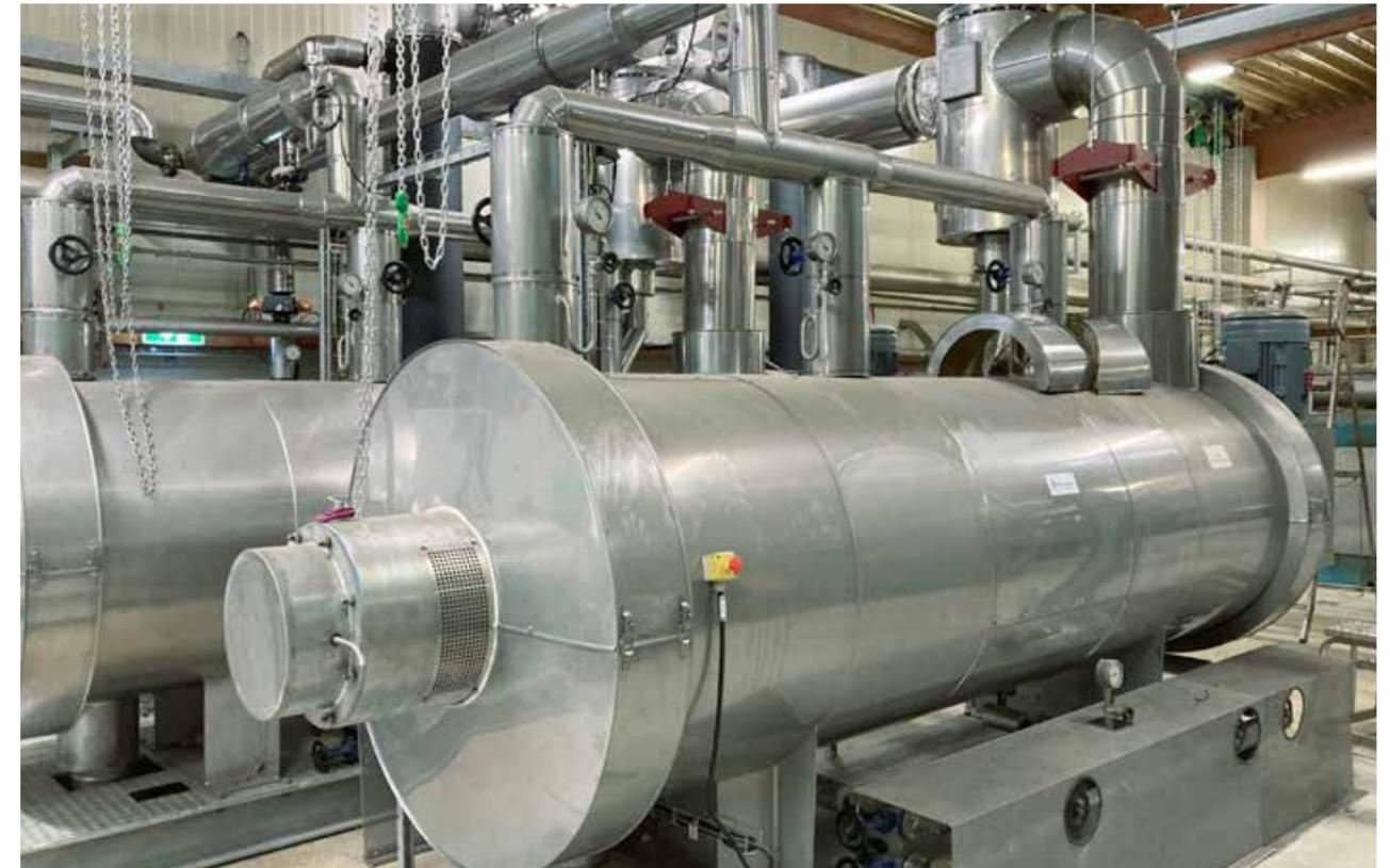
The two thin-film dryers are installed in parallel at Power Oil Rostock. © GIG Karasek
