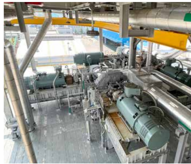
Example: Industrial heat pump solution with Piller compressors (GIG Karasek offers compressors from various OEMs). © Piller
